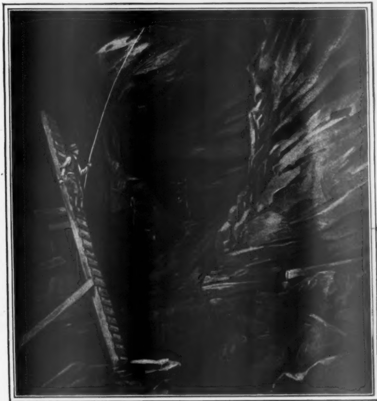
"WHERE A FIRE OF GAS, GENERATED AND LIGHTED BY BURNING COAL, BURNED OUT A FORTY FOOT DOME IN THE SOLID ROCK."
